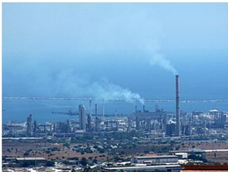
Figure 1. Augusta-Priolo oil refinery plant.
